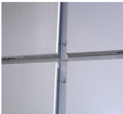
Obr. 15 Detail spáry.
